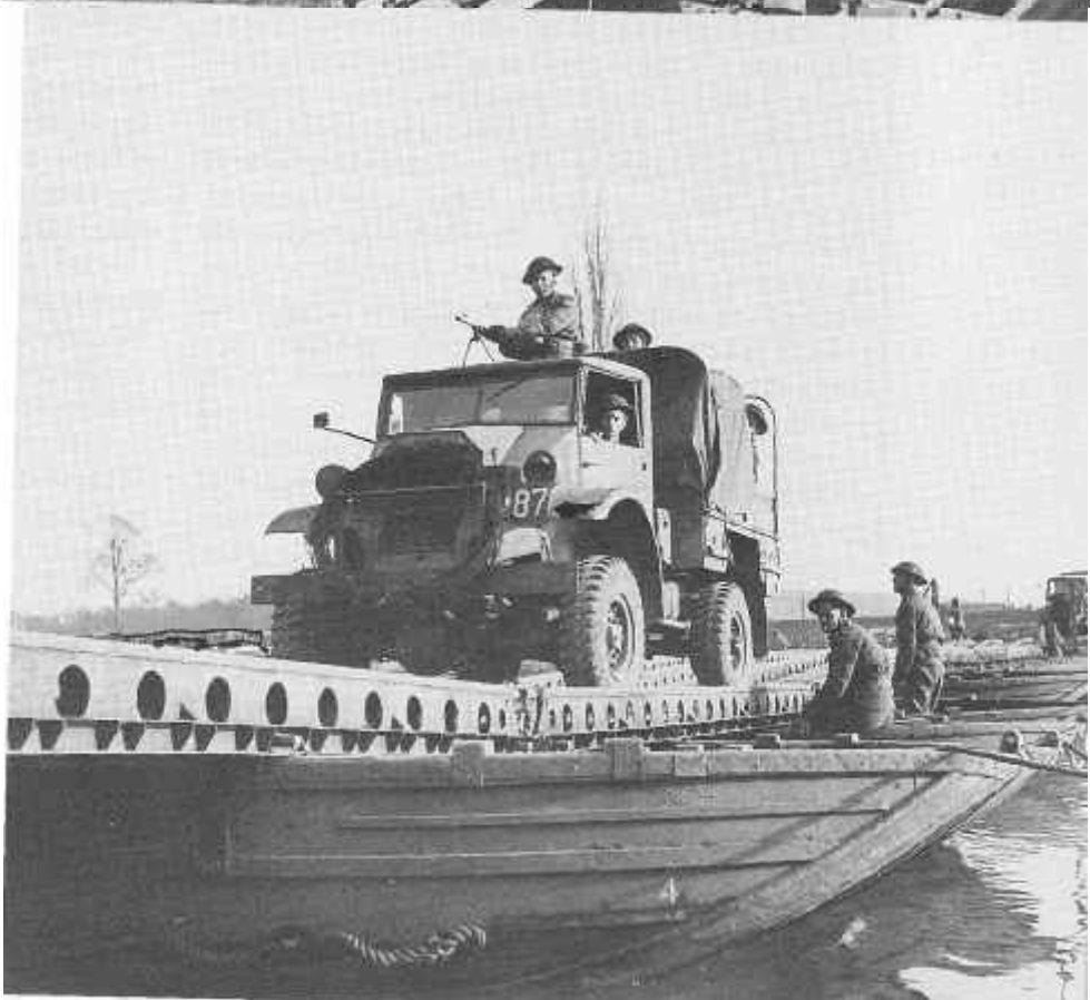
Top: Canadian Engineers of I Canadian Corps work to assemble a pontoon bridge across an English river during Exercise "Spartan." Theoretically, the permanent bridge was "destroyed."
