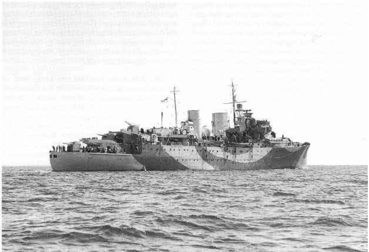
Aft view of HMCS Prince Robert in 1943. The three twin 4-inch gun mountings of the aft group are clearly visible. (NAC PA 145618)
