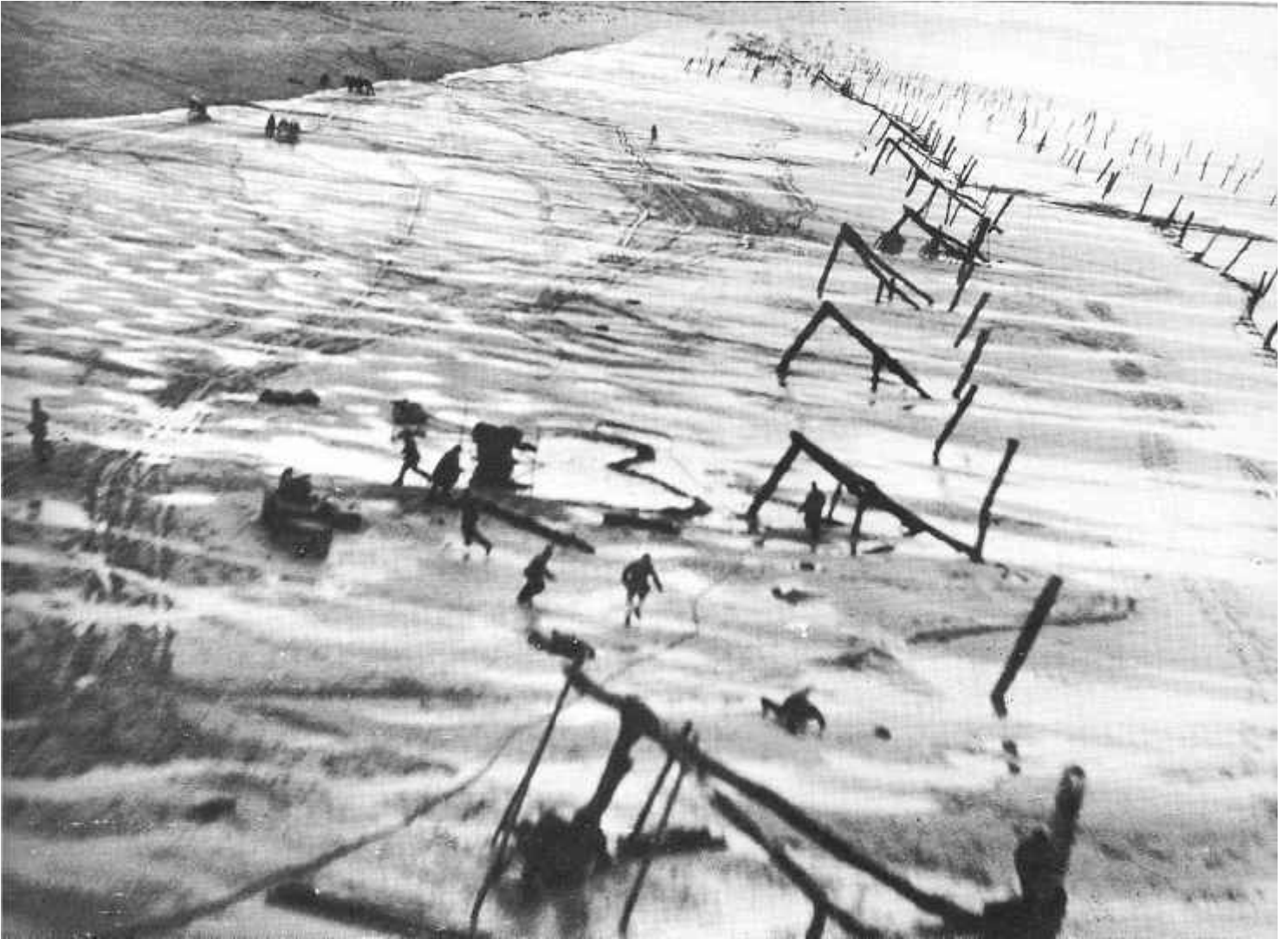
A reconnaissance flight over the Normandy beaches on 6 May 1944 catches German troops scrambling for cover. Detailed information on the beach defenses was obtained from "dicing" shots like this one. Timber ramps, with mines or saw-toothed blades to take out the bottoms of landing craft, are clearly visible.
